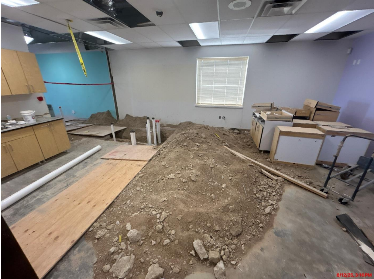
Under-Slab Plumbing Work
